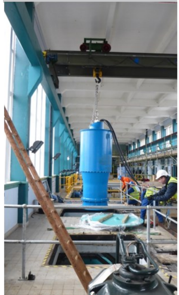
Bedford Pumps SAF pump being installed at Crossens
