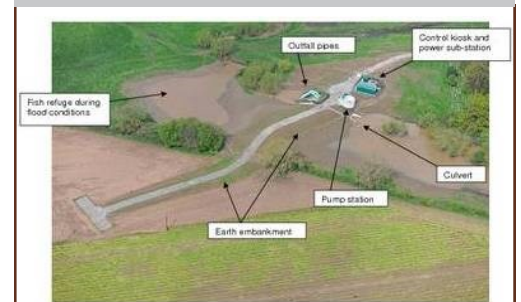
Flood Risk Management Scheme
