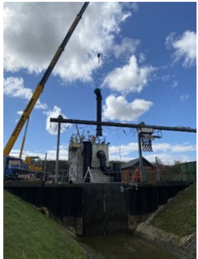
Fig 2. North Lynn Pumping Station
