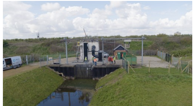
Fig 1. North Lynn Pumping Station
