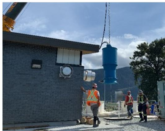
*Fig 2. Fish Friendly pump installation at Pitt Polder P.S.*
